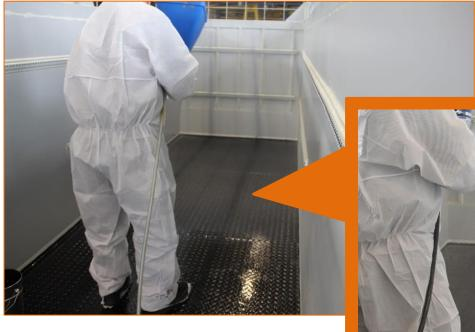
7. Apply LOGIS GRANOFLOUR (Sanding) with a funnel gun on the damp floor.
