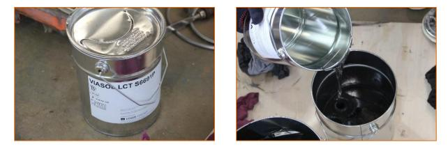
4.3 Stir both components well together (approx. 2 min)
