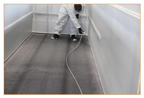
As soon as the surface is free of adhesive, the fabric adhesive tape should be removed. Curing time until full load approx. 8 hours.
