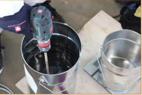
4.2 Then fill 50 parts B component into 100 parts A component
